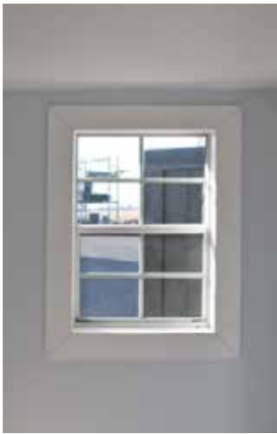
R-11 Insulated w/ Trusscore Lined Interiors
